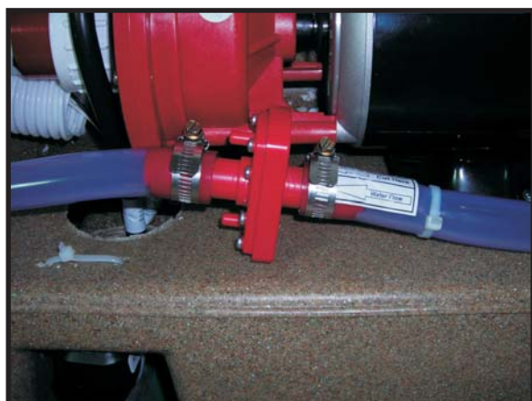
3. Install ozone injector between the cut hoses. Make sure that the flow arrow is pointing towards the INLET side of the injector.
