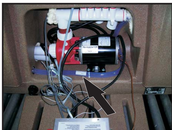
1. After disconnecting power to spa and removing all the water, open equipment door and locate the ozone injector hose.
